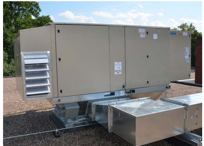
Left: Egan Company installed Daikin Applied’s highly efficient Rebel rooftop units to meet the dehumidification challenges faced by two Bethel University residence halls due to showers, open doors, and a variable Minnesota climate.
