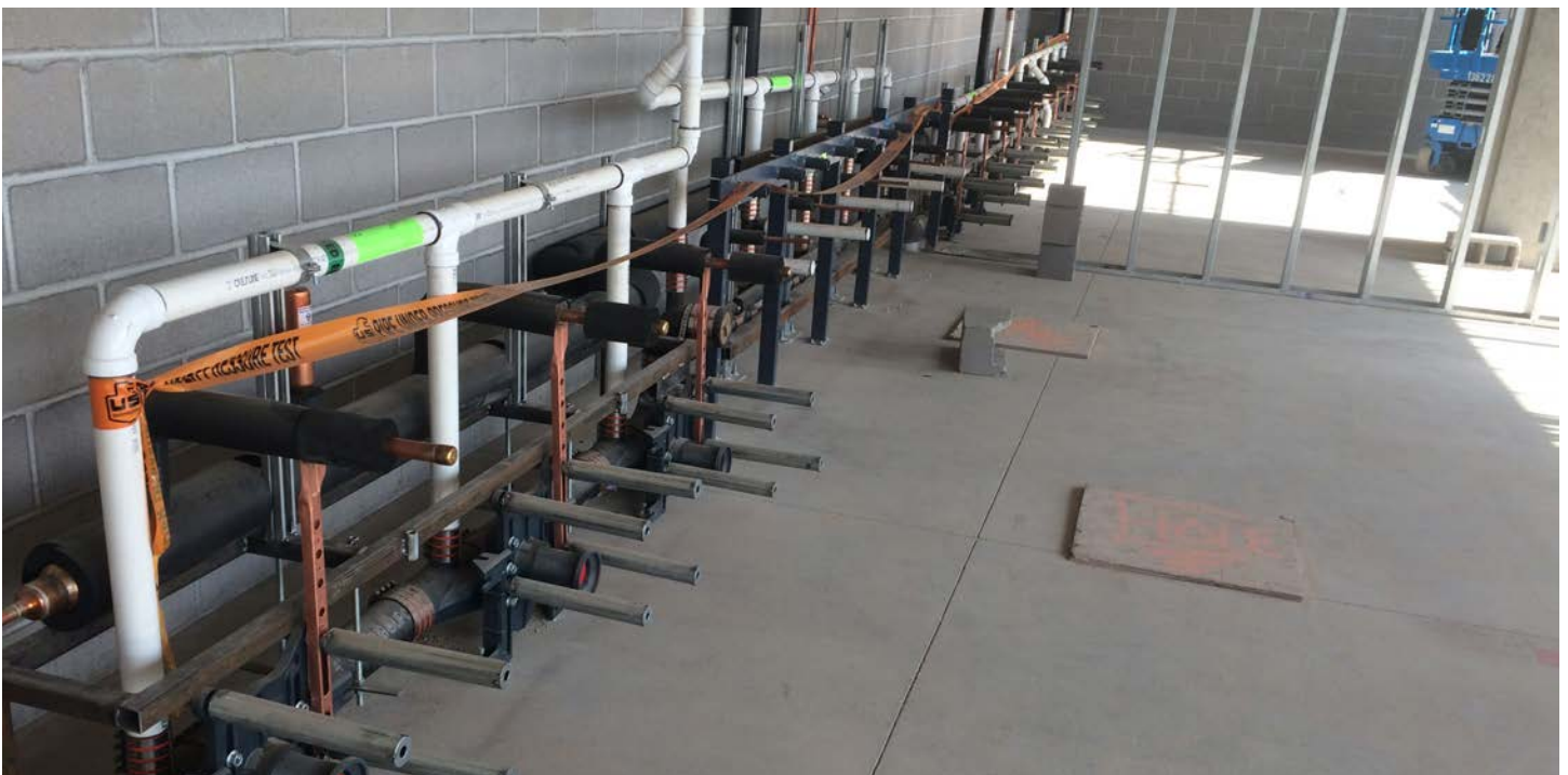
Zurn custom built lavatory and urinal carrier banks (Z1231-CB and Z1222-CB) designed to fit predetermined spaces, so U.S. Engineering only had to do “quick adjustments” rather than building and setting each carrier.
