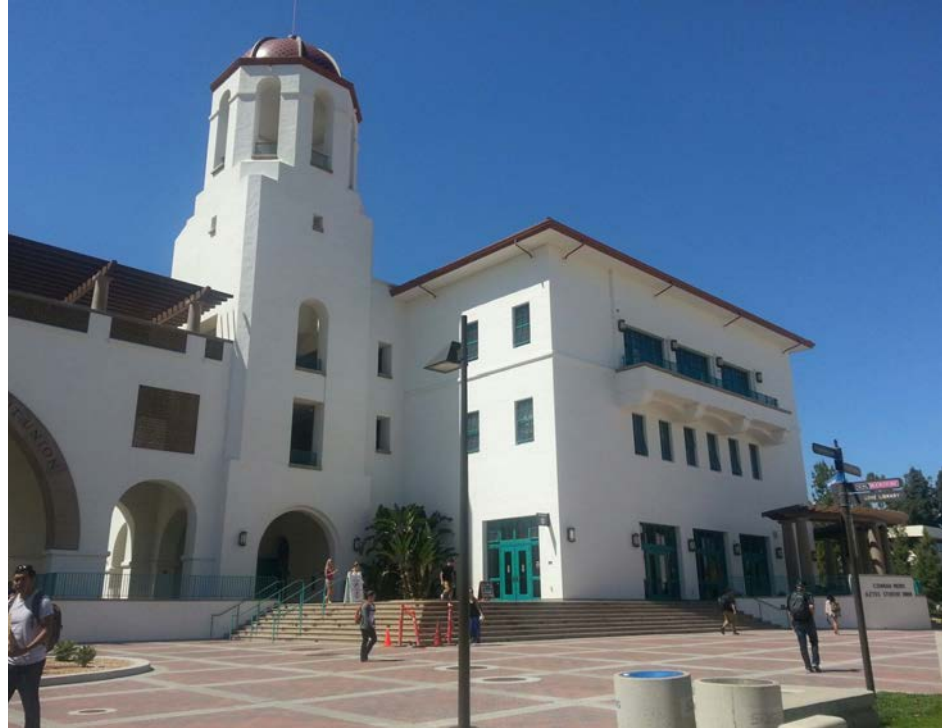
University Mechanical helped San Diego State University's new student union reach LEED Platinum certification with sustainable, energy-efficient solutions like Uponor's radiant heating and cooling.
