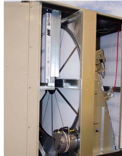
Egan Company found the Daikin Rebel rooftop unit improved student comfort and delivered substantial energy savings thanks to an energy recovery wheel that draws 60 percent more humidity from the air stream.
