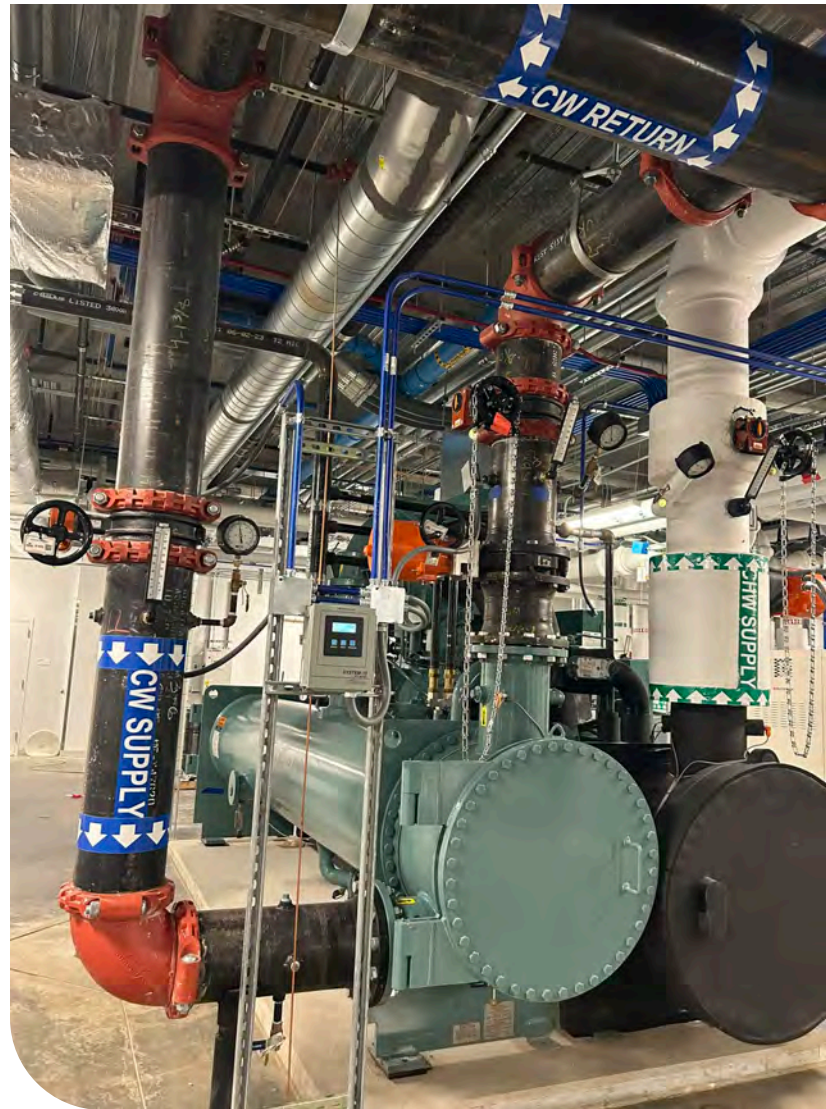
Heffron Company strategically placed flexible Victaulic couplings to accommodate movement within the piping system of a cutting-edge life sciences facility, eliminating the need for expansion loops.
