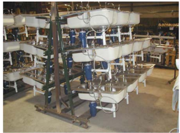
Custom carriers are a valuable way to store, transport and install prefabricated assemblies onsite. Photo courtesy of the P1 Group.
