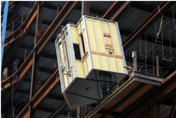
Module Being Hoisted up for Installation
