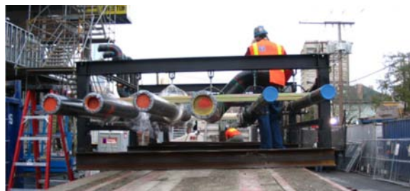
A pre-fabricated rack arriving on a jobsite.
